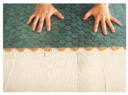
STEP 2: Sheets are face-mounted. Carefully place the Cork Mosaic with the plastic sheet facing upwards, contacting the backside of the sheet to the adhesive surface.
