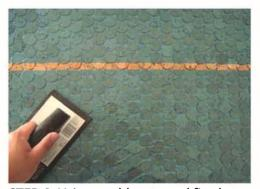
STEP 4: Using a rubber trowel firmly press against all areas of each Cork Mosaic sheet. This is important to obtain proper contact of the material and adhesive surface.
