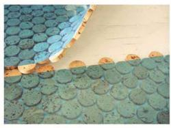
STEP 3: Interlock and aligh each Cork Mosaic sheet carefully next to one another. The material can be easily cut and shaped using a utility knife.
