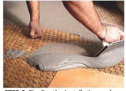
**STEP 6:** Finalize the installation and using a high quality rubber trowel, apply tile grout. We recommend the use of a polymer modified sanded grout or premixed quartz or urethane. (Mapei, Laticrete, Bostik Trucolor, Custom Fusion or Litikol)
