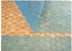
**STEP 5:** Following adhesive instructions, and once fully dry. Carefully begin to peel off and away the plastic face mounting and discard. If necessary, re-attach any loose cork chips manually.
