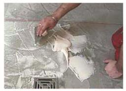
STEP 1: Apply a uniform layer of tile adhesive using a V-notch trowel (3 mm) Note: most common thin-set mortar adhesives are suitable for Cork Mosaic. (i.e. Mapei, Custom, Laticrete, Litikol)
